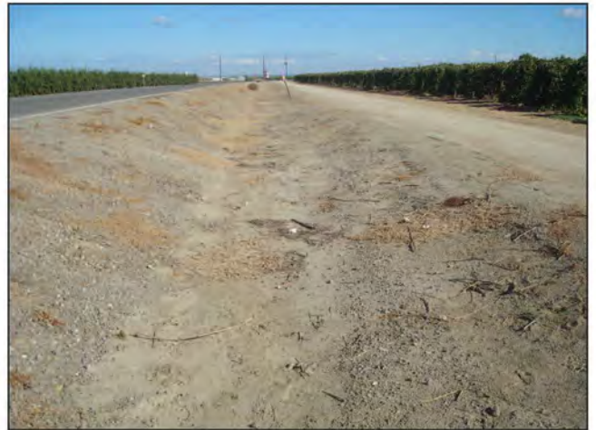
PHOTO 5: View of drainage ditch and access road along Wheeler Ridge Access Rd facing north.
