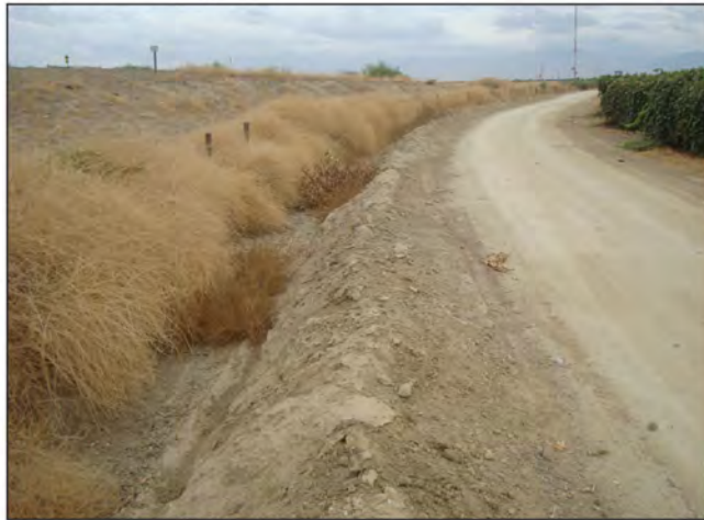
PHOTO 3: View of drainage ditch and access road along the north central boundary of the project site facing east.
