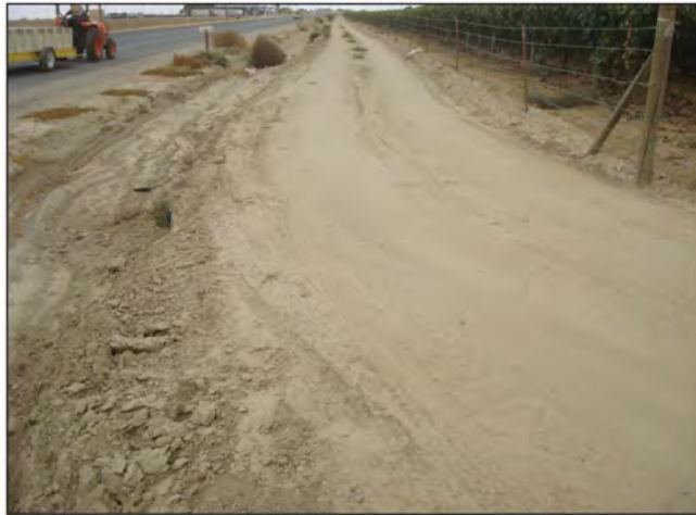
PHOTO 1: View of drainage ditch, access road and agricultural vine rows along SR-166. Photograph taken from the northwestern corner of the project site facing east.
