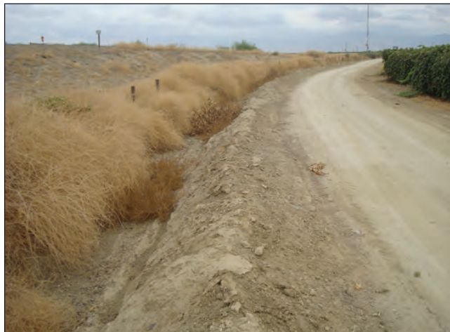
PHOTO 3: View of drainage ditch and access road along the north central boundary of the project site facing east.
